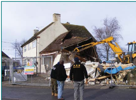
The shop being demolished
