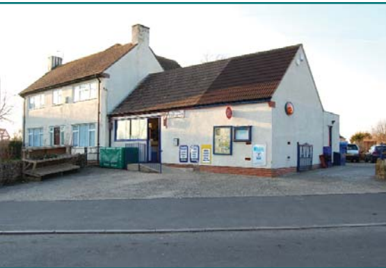
The extension has different colour roof tiles
